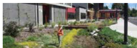
A Stormwater Bioretention facility in Olympia.
